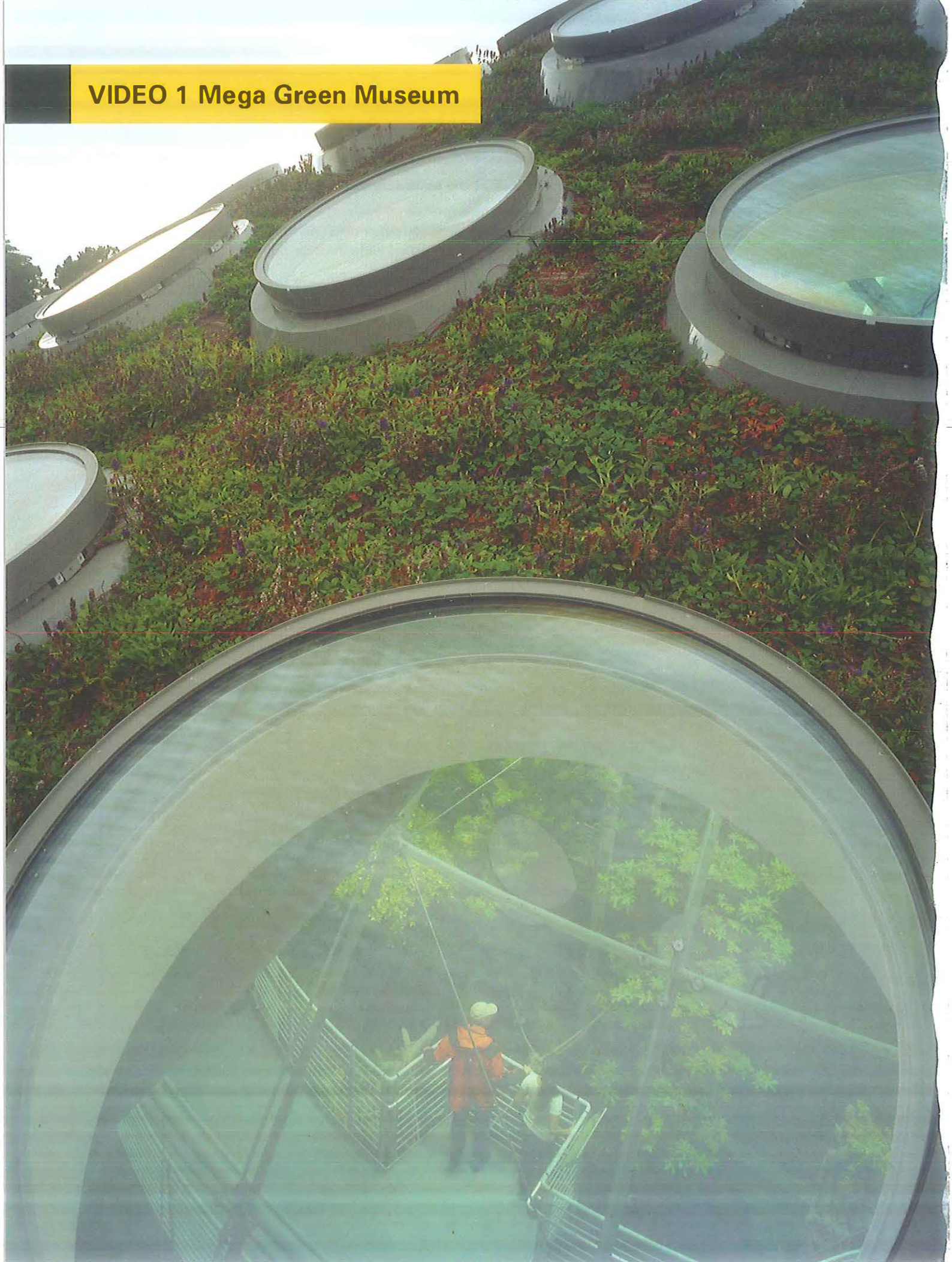
Skylights on the roof of the California Academy of Sciences Natural History Museum
